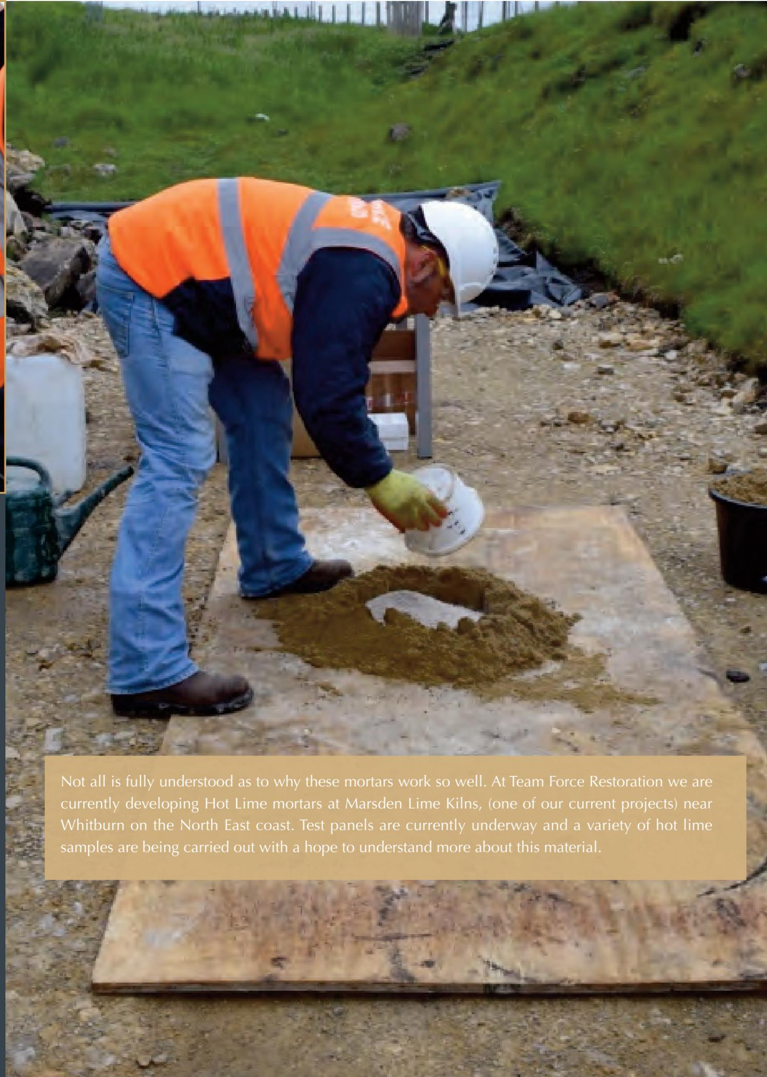
Not all is fully understood as to why these mortars work so well. At Team Force Restoration we are currently developing Hot Lime mortars at Marsden Lime Kilns, (one of our current projects) near Whitburn on the North East coast. Test panels are currently underway and a variety of hot lime samples are being carried out with a hope to understand more about this material.
